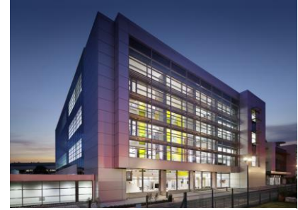
The Etherow Building
